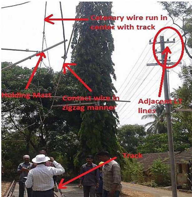
Fig. 7. Experiment conducted on a 50-m-long prototype of conventional OHE.
