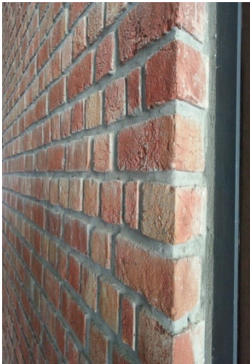
Fig. 5. (a) Walls with Proper Finishing
