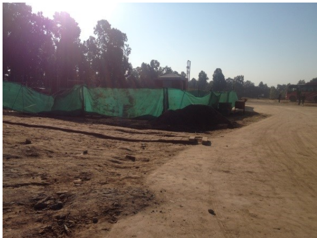
Fig. 2. (a) Barricading Near the Path Way
