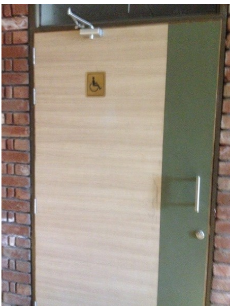
Fig. 4. (a) Rest Room Facility
