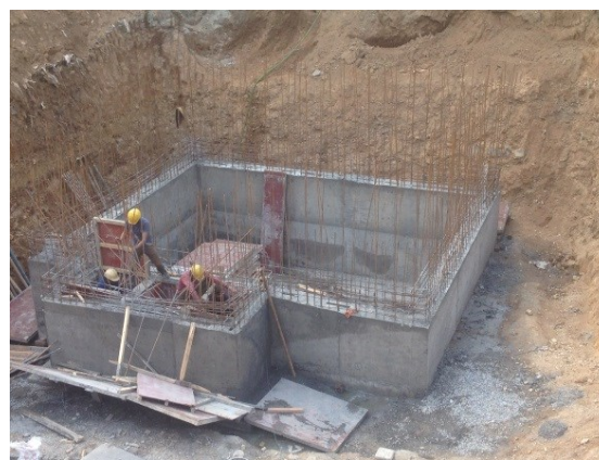
Fig. 3. (a) Construction of STP
