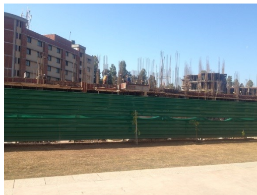
Fig. 2. (b) Barricading at Construction Site
